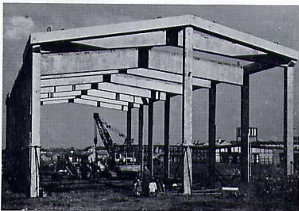
NEW CHURCH IN COURSE OF ERECTION.
